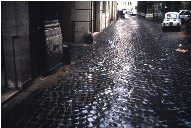
The old streets of Rome are paved in blocks of black basalt. When these are set on the diagonal, which distributes the stress of wheels more evenly.
